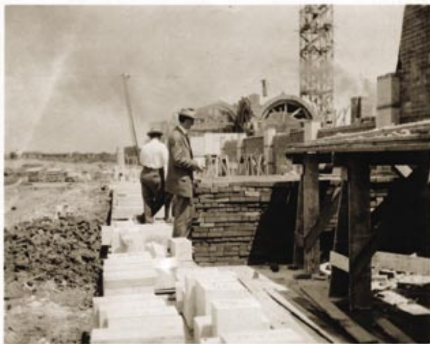
Architect William Ward Watkin examines a test on a cloister slab for the Administration Building (now Lovett Hall).
