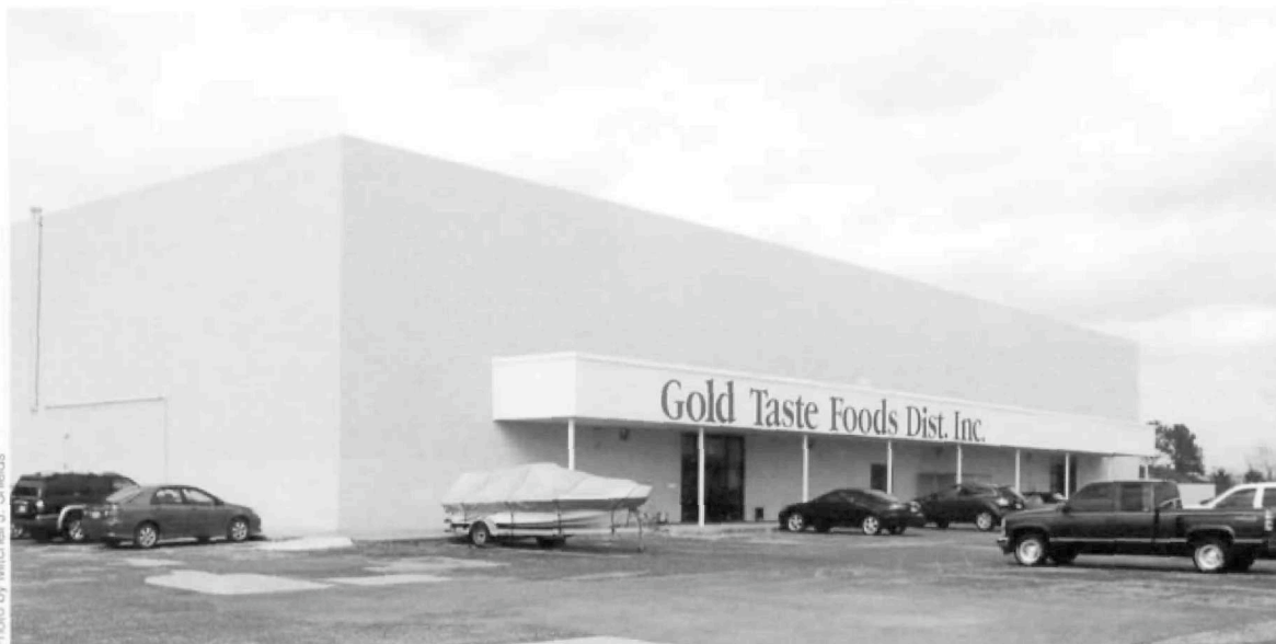
The BEST Products building at three stages of its life. Top: With original façade intact. Center: After façade's removal. Bottom: As it is today.
