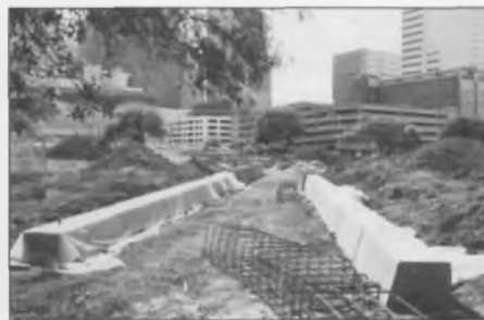
Walkways take shape at downtown's Market Square Park.
